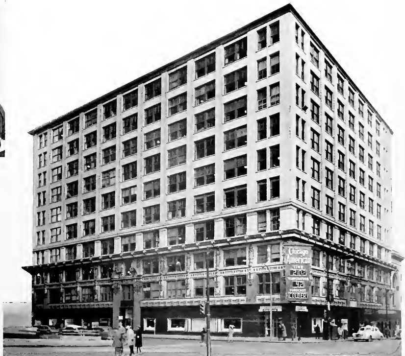
Headquarters for the Chicago American is the American Building , located at 326 West Madison.
